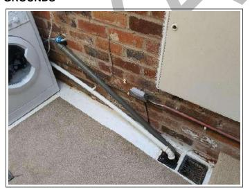
**CONDITION SUMMARY:** There are PVC grey water pipes that appear to be in a reasonable condition. The grey coloured pipe may require bracket to help prevent it from disfiguring.
