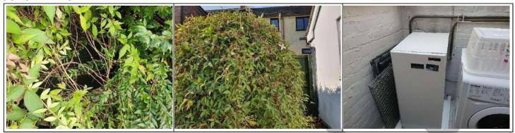
**CONDITION SUMMARY:** The oil tank is located in the grounds to the rear. The location of the tank does not appear to be compliant with safety regulations. The tank is also covered by a large Vine. You should discuss this with an OFTEC registered engineer. The oil fired boiler is in the front porch and appears to be old full. The boiler could require replacing soon and they should be discussed with your Engineer.
