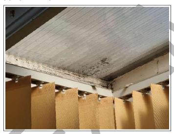
**CONDITION SUMMARY:** Some deterioration appears to be occurring to the wall plate of the front porch. This has probably been caused by condensation or excessive water not reaching the rainwater fittings externally. This should be discussed with the contractor who repairs the roof panels.
