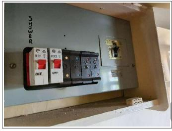
**CONDITION SUMMARY:** There is an old rewireable type fuse board still in place in the kitchen. This is considered to be a Health and Safety risk. An Electrical Installation Condition Report should therefore be obtained from a qualified electrical contractor and all recommendations implemented.
